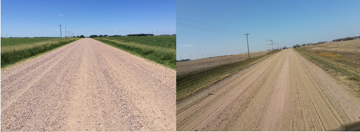
Figure 49 Seven Months after Construction-Jackson County
