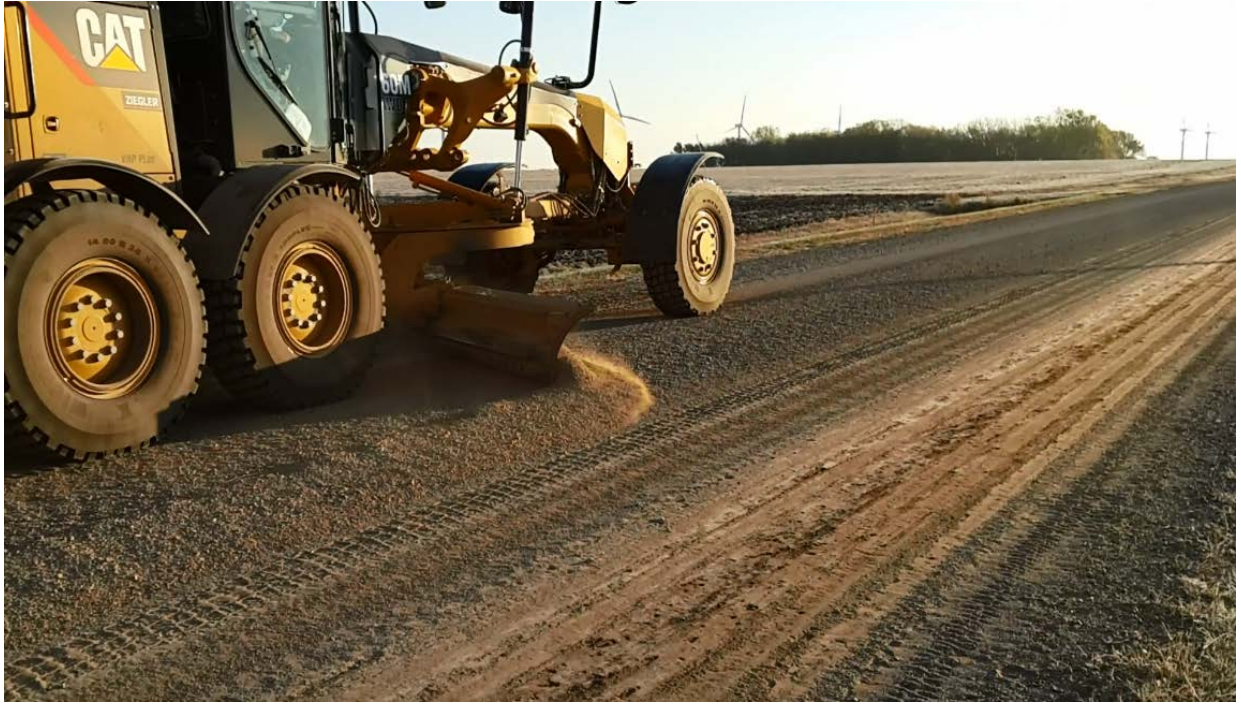
Figure 25 Surface Gravel Windrowing (Photo by the Author)
