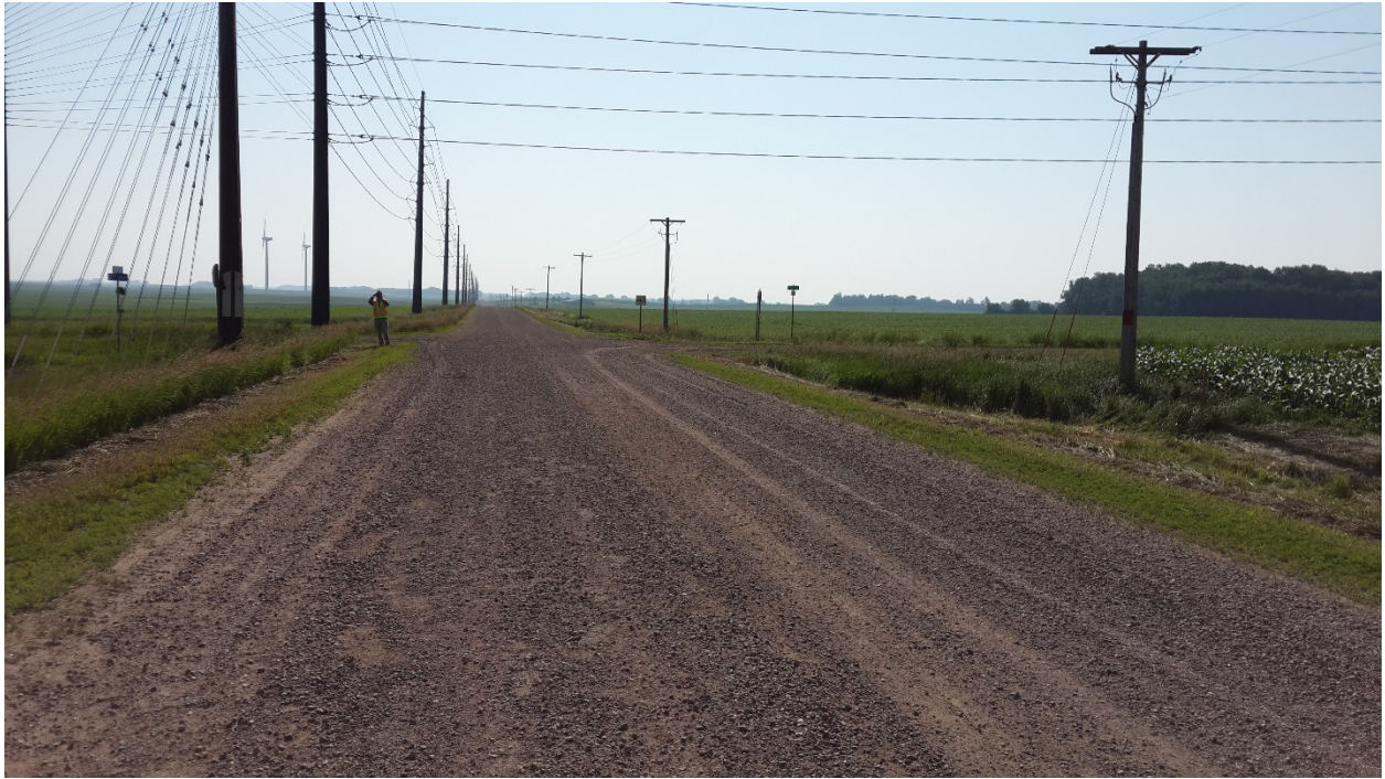
Figure 21 Jackson County Road 76 Surface Conditions in July, 2013 (Photo by the Author)
