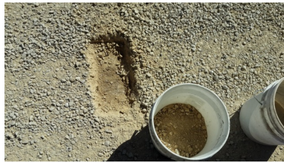
Figure 15 Bottom Compacted Aggregate Collection (Photo by the Author)
