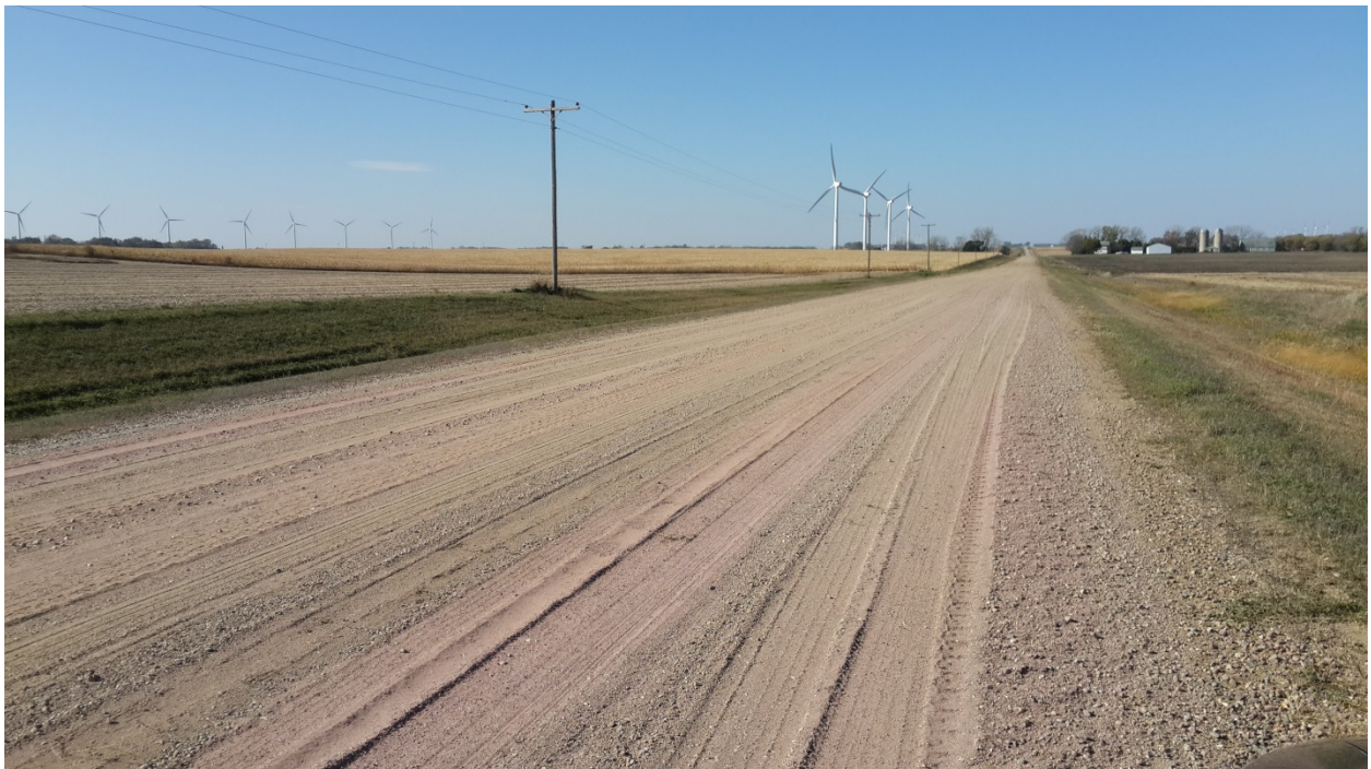
Figure 29 Jackson County Road 76 Mid Test Section (Photo by the Author)
